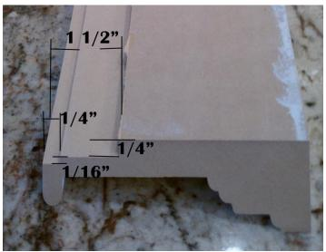
5. Assembly time: Make sure the bottom rail (with only one rabbet joint) goes on the bottom. Try not to get glue in the rabbet joints (grooves) where the pictures slide. Using the following dimensions and wood glue, glue and clamp each rail and top moulding in place. Allow glue to dry, minimum 1 hr.
