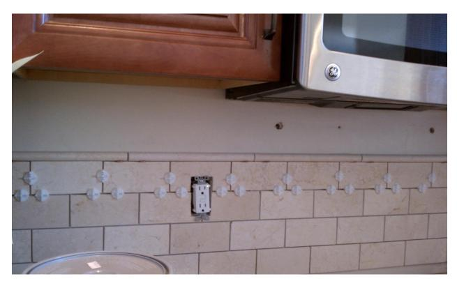
Applying the glass mosaic is simple. Spread mastic on the wall and use the trowel to make the grooves. Lightly press the sheets of mosaic onto the mastic. When you reach the end, you can cut the mosaic with the tile saw.
