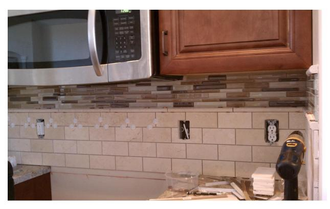
Clean up any extra mastic that might stick up above the grout. Allow the tiles to cure for 2 days. Remove all of the spacers/pennies.
