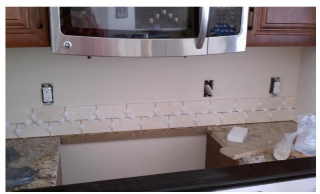
Continue the pattern, when you come to an outlet, cut the tile accordingly. I learned a little trick for cutting a U out of a tile. Approximately trace the outlet box on the tile, cut along the side lines, make additional cuts about ½"-1" wide. Knock out the inner pieces. Most of the time it'll make a straightish
