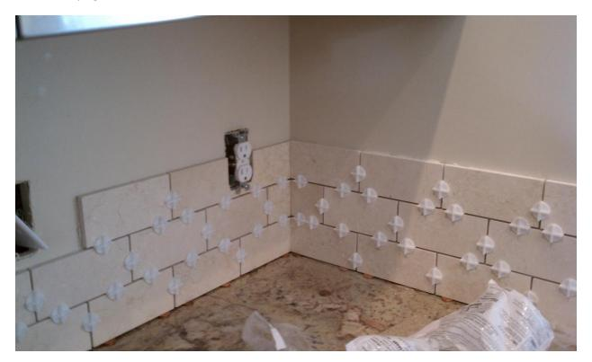
I used a travertine bull nose trim to separate between the travertine and glass mosaic.
