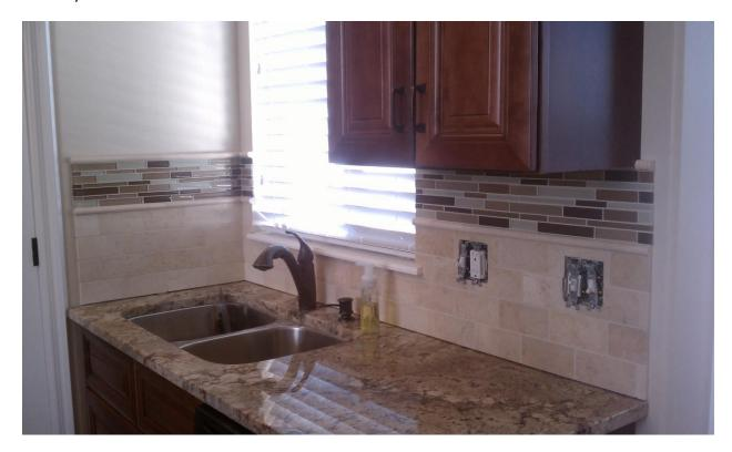
Use unsanded grout caulk, same color, and run a bead of caulk between the counter and bottom row of tile. Also run a bead on any vertical exposed surfaces and corners. Use a wet finger to get a smooth finish on the caulk, and a wet sponge to remove excess. Allow the caulking to dry.
